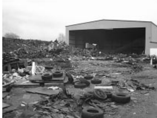
Abandoned, unpermitted recycling facility
