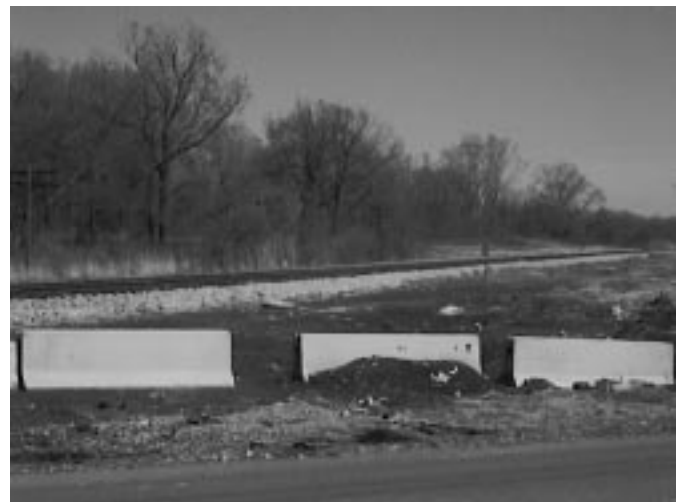
Concrete barriers preventing access along railroad right-of-way
